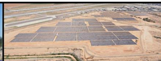
Luke AFB – Solar Facility
