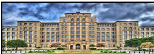
JBAS – Old BAMC Office Space Renovation
